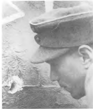
A Luftwaffe officer inspects the pierced 78-85 mm thick cast turret side of a T-34.
